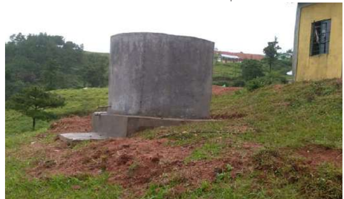
The tank constructed at Laitsohpliah RCLP & UP School.
